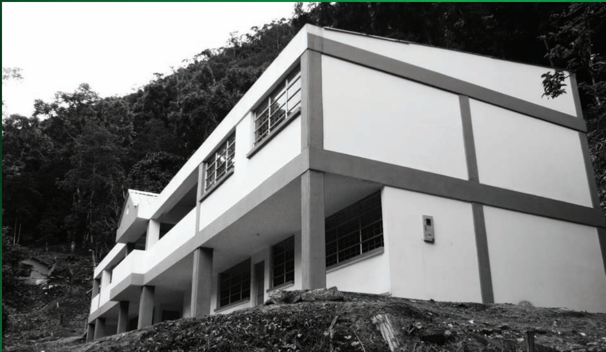
The newly built school in Muzo, Colombia.
